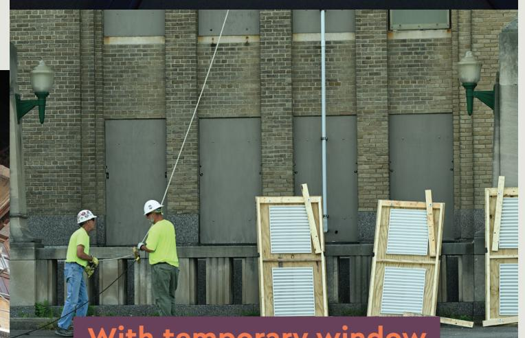
**With temporary window coverings in place, masonry repairs can begin.**
