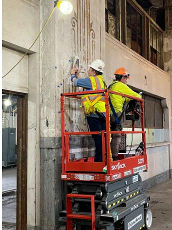
Figure 20: Testing of decorative finishes in Restaurant by project conservator, Stephanie Hoagland, Jablonski Building Conservation. (Courtesy BAC/Architecture + Planning, PLLC)
