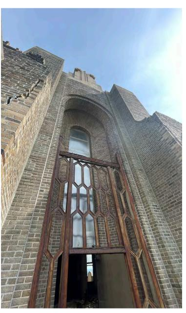
Figure 185: Buffalo Central Terminal, Penthouse floor, on balcony looking up at cast iron grille and window, July 2023. (Courtesy BAC/Architecture + Planning, PLLC)
